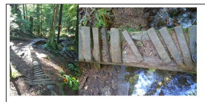
Describe Problem: The entrance of the ladder bridge is missing rung's and the stringers are rotting hemlock. The span across the creek is missing some rungs.
