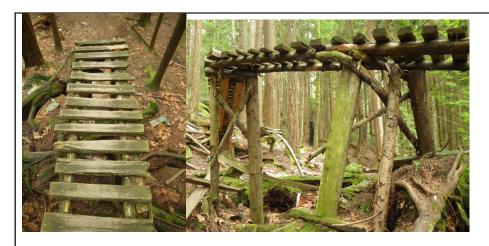
Describe Problem: Stringers on the original section of the pile driver are in need of replacement as well as some of the support posts
