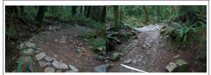
Describe Problem: A number of the larger berms are poorly aligned, not round making sharp angles. The berms are also incomplete, not finishing off onto the ground.
