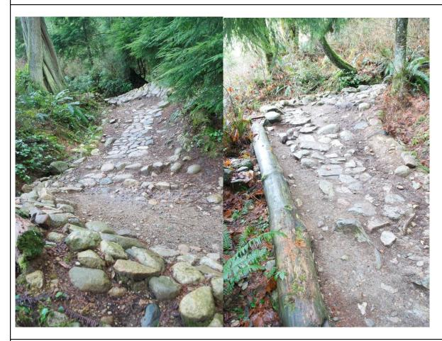
Describe Problem: Rocked berms that have eroded out due to rider use and sediment removal from surface run-off. There are 10 berms of this type that will require maintenance.
