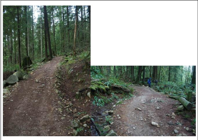
Describe Problem: high-speed area above blind junction with Empress (left). Trail erosion on trail sides and lack of ecologically balanced vegetation in area. Widened trail base does not give rider clear visual line of alignment.
