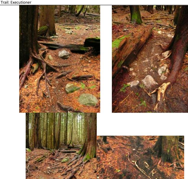
Describe Problem: tree roots, mostly Cedar, are exposed and being damaged on old & new alignments of the trail Solution: build rock and mineral dirt over top of roots, use cribbing where necessary to create a raised trail bed
