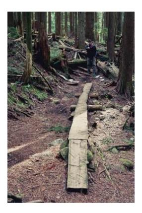
**Problem:** Woodwork is in poor condition. Ripped wood is very slick when wet thus increasing rider
