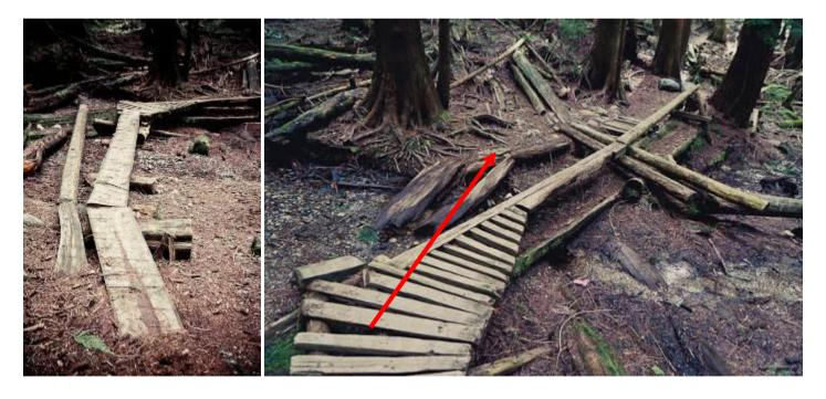
**Problem:** Wood work is near expiry, off cambered and ripped wood is very slick when wet thus increasing
