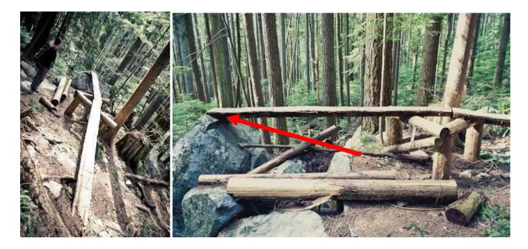
**Problem:** Structure will eventually fall apart and the skinny is planed wood which is slippery when wet. **Solution:** Remove first section of structure. Create a wooden frame (where the red arrow is) with existing material and fill in with rock and top off with gold.
