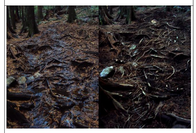
Describe Problem: Braided creek above runs onto eroded trail bed in several spots and is trapped for approximately 100+ feet. The area has been severely eroded and the alignment runs close to trees, therefore exposing root systems.
