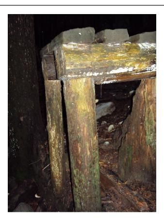
Describe Problem: Wood structure is beginning to rot as evidenced with cracking of stringer and fungus starting. The platform drop is at the end of a high speed fall line section - the stunt doesn't match the entry speed and riders overshoot to land on flat area without transition.
