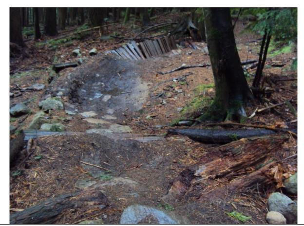
Describe Problem: Water is trapped in low area. This section has a poor user experience and the combination of speed into a sharp turn further impacts the low drainage area with braking forces.
