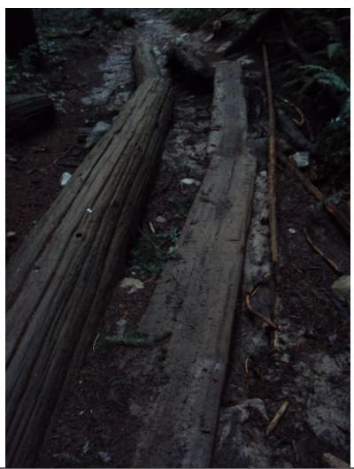
Describe Problem: This section is misaligned and the woodwork slippery. Combined with the fact it is a high speed section requires a solution to mitigate risk.
