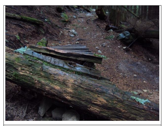
Describe Problem: Stunt has twisted over time and is off camber in the middle of a high speed section.
