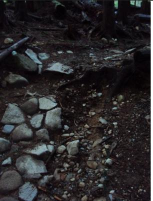
Describe Problem: Entrance is severely eroded and straight fall line requiring heavy braking which further degenerates the heavily eroded trail bed. Old armouring is chunky and has shifted over time making navigation a challenge. User experience is poor and riders are creating a new loam entrance.
